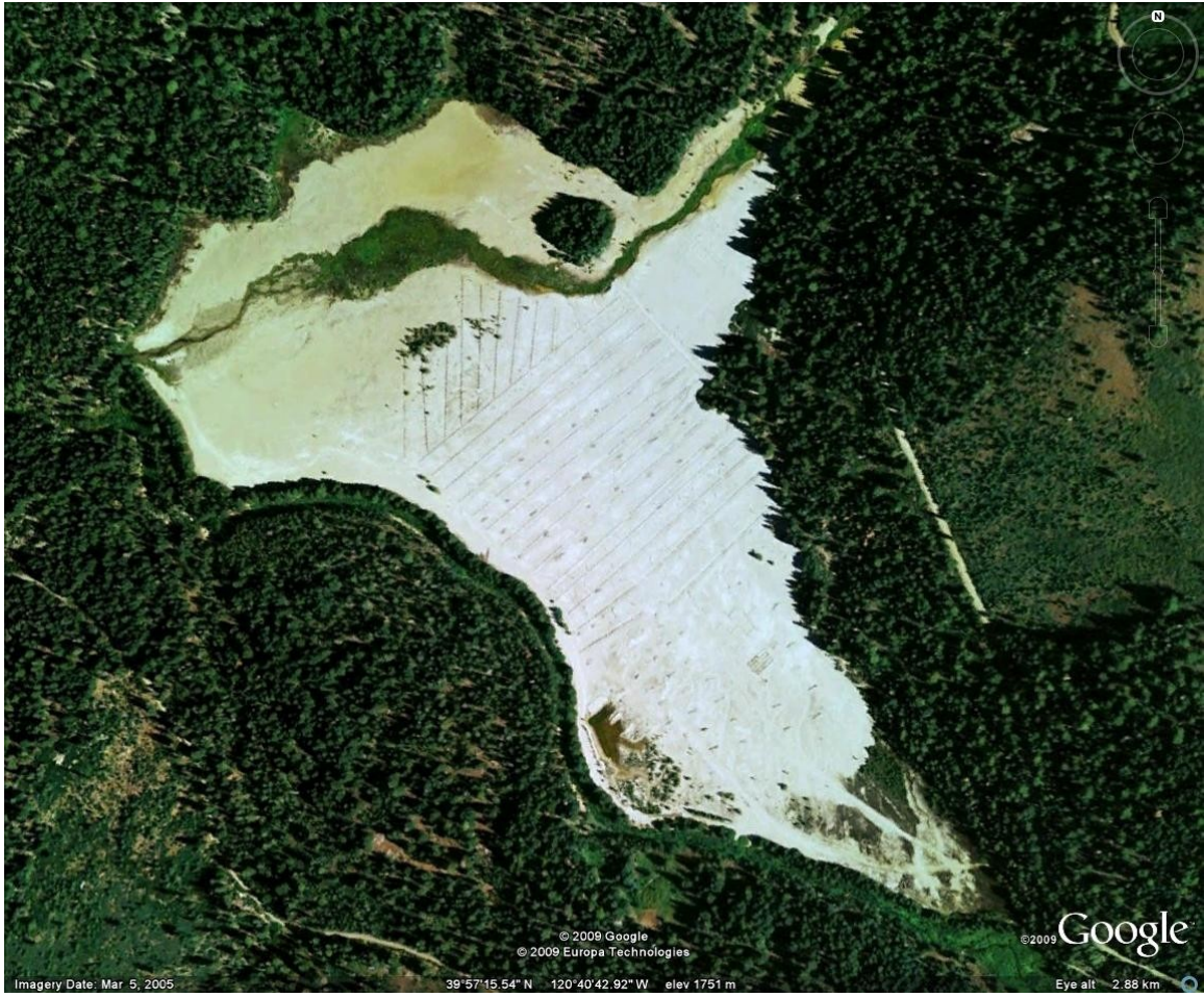
Walker Mine Tailings project
